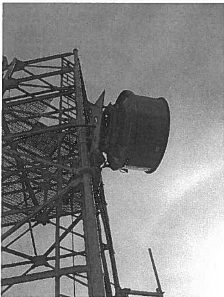
Figure 3. Peak Signals technician aligning high wind-load microwave antenna.
