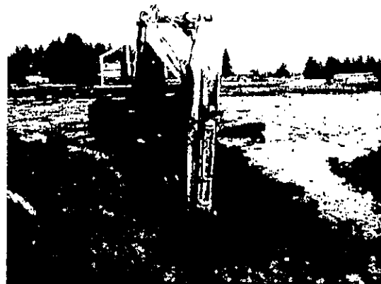
Photo 2: Excavating into glacial till at TP1.
