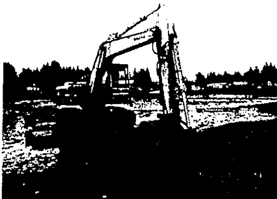
Photo 5: Excavating through surface horizon of silty sand at TP2.
