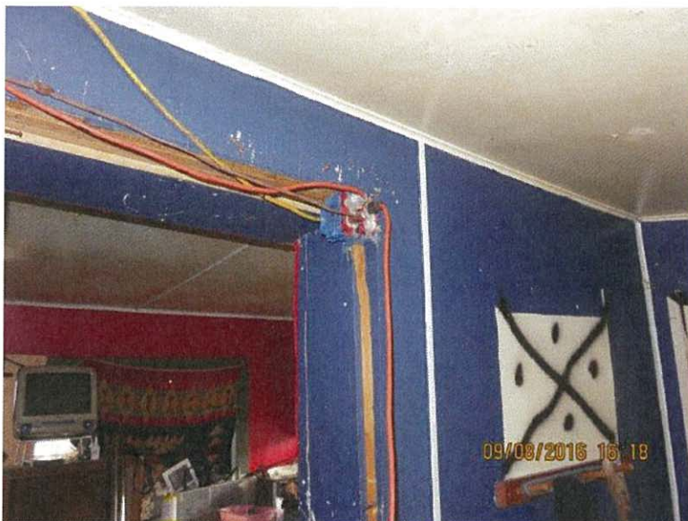
Extension cord spliced into box with additional cords plugged in.
