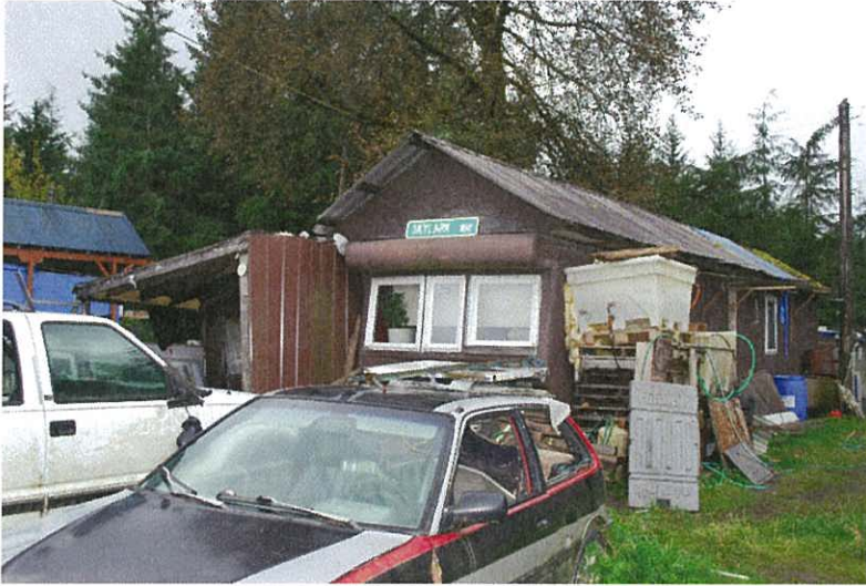
Exterior of structure
