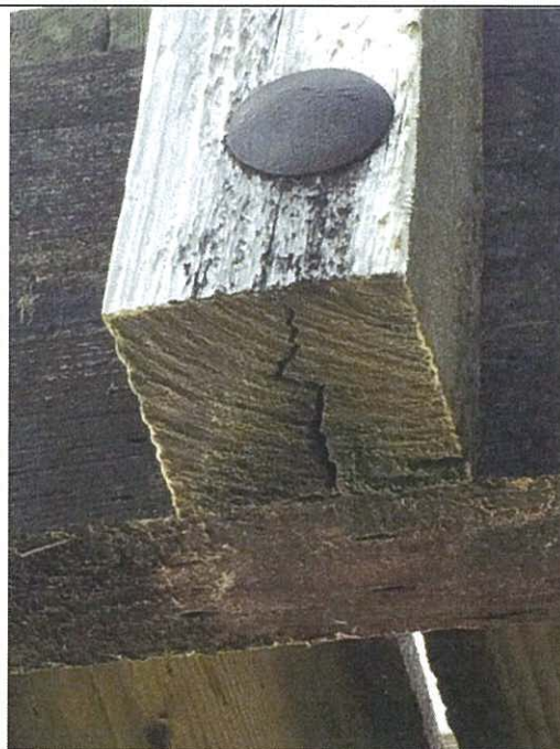
4. Typical Crack at Handrail Post
