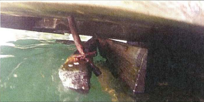
9. Damaged bullrail and lip at float intersection
