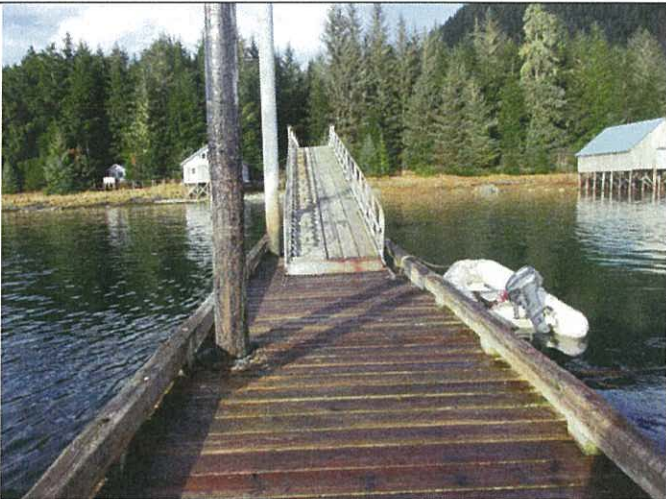
5. Hollow Approach Bearing Pile
