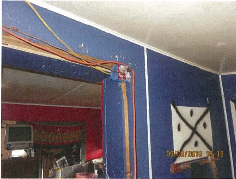
Extension cord spliced into box with additional cords plugged in.
