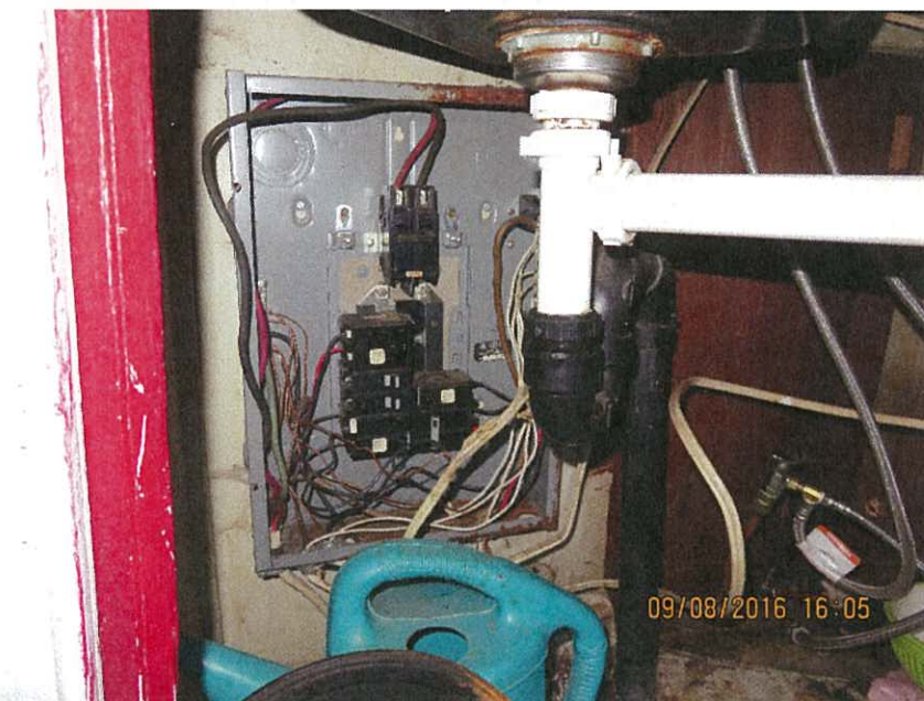
Compromised breaker box under sink.
